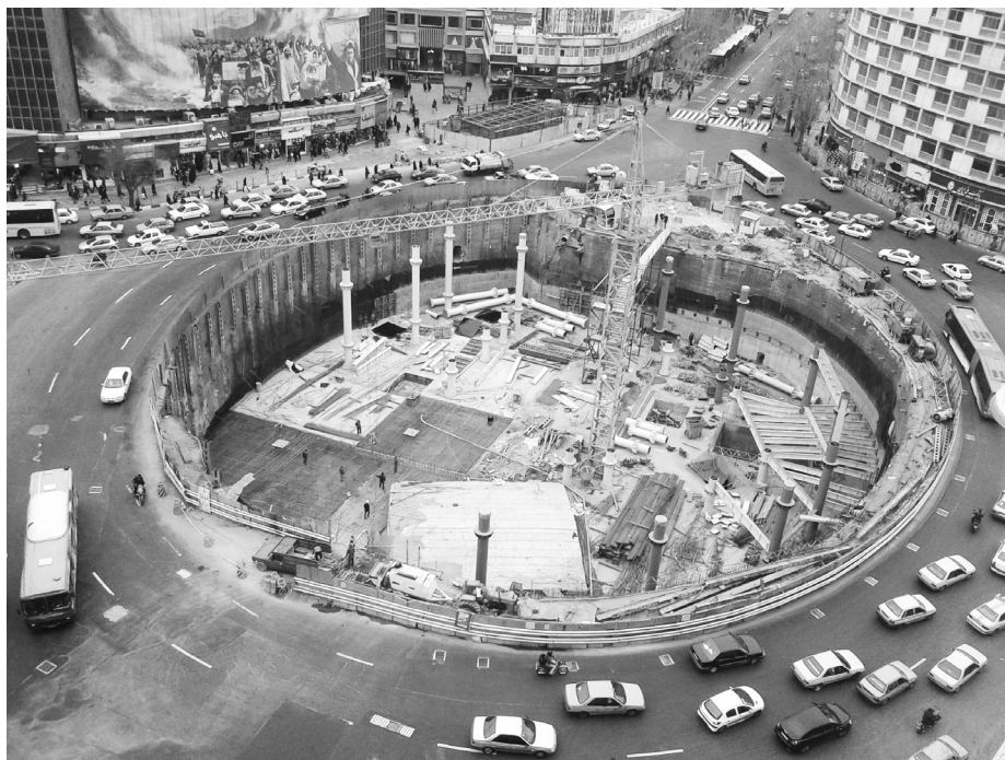
Line 3 of Tehran Metro - Vali-e-Asr Square Plaza-Station ▲
